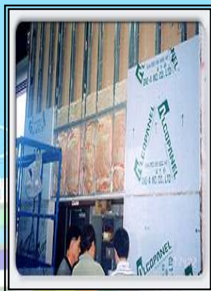
2. The Alcopanel/fr, Exterior Wall System Construction
